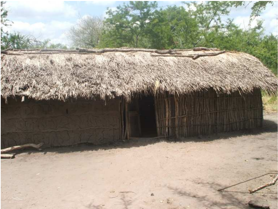
Figure 13: Traditional Maasai home built from a wooden frame and then covered in mud. Source: Allison Kotowicz, 2012.
